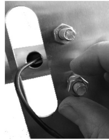
b) Fix the pipe with the two brides. Take care at the antenna cable which must pass through the ovale hole.
